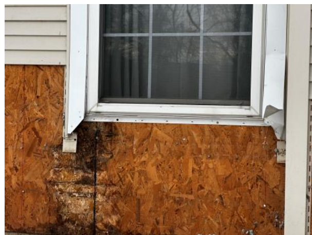
Photo #76: Overview of existing sheathing in poor condition below a lower window at Unit 12.
