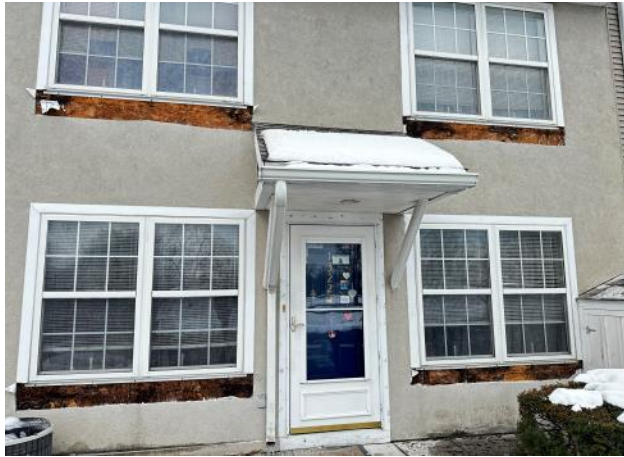
Photo #93: Overview of existing sheathing in poor condition below the four windows at Unit 1322.
