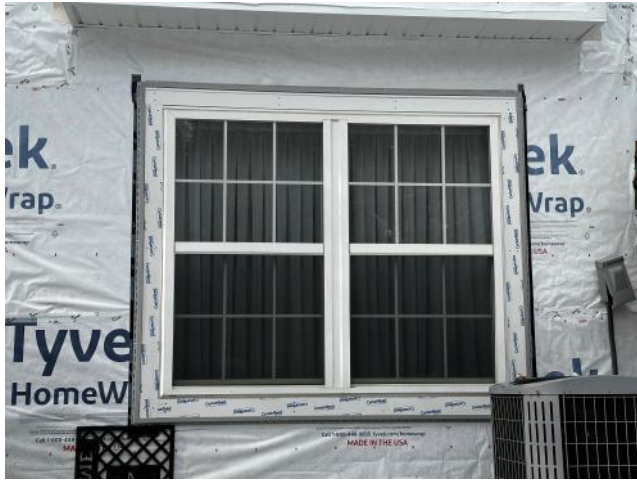
Photo #29: Overview of new pvc trim installed at a window.
