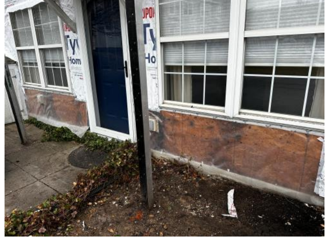
Photo #82: Overview of existing sheathing in poor condition below lower windows at Unit 27.
