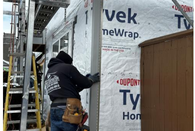
Photo #62: Overview of a new vinyl corner being installed.
