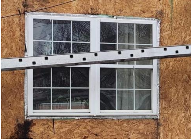
Photo #85: Overview of existing sheathing in poor condition below a lower window at Unit 25.
