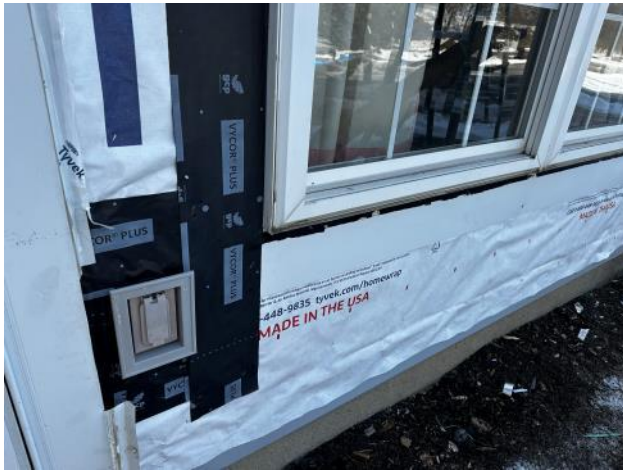
Photo #7: Overview of metal flashing installed at the bottom of a window and flashing tape installed as well.
