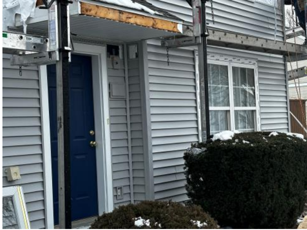
Photo #65: Overview of new vinyl siding being installed.
