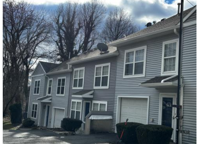
Photo #4: Overview of new vinyl siding installed at a front section of Building 5.
