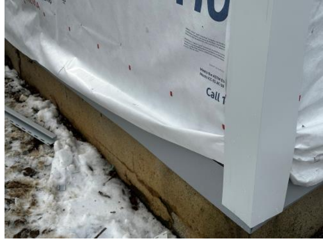
Photo #30: Overview of new starter metal flashing installed.
