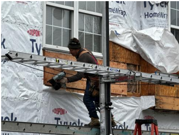
Photo #51: Overview of new sheathing being installed.
