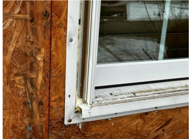
Photo #46: It should be noted that windows at Unit 31 were observed no to have a proper window flange.
