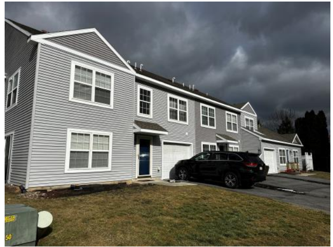
Photo #14: Overview of new vinyl siding installed at a front side of the Building.
