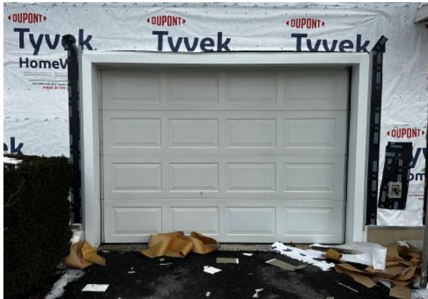
Photo #61: Overview of a garage door frame properly flashed.
