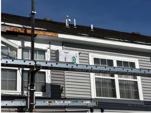
Photo #33: Overview of new intake soffit being installed.
