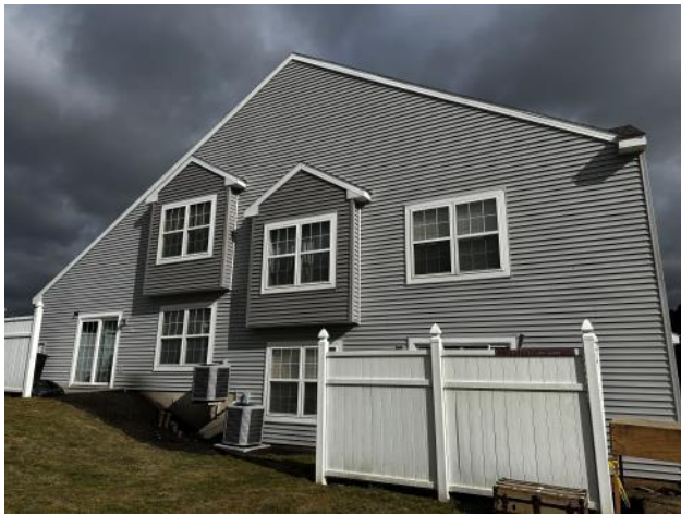
Photo #15: Overview of new vinyl siding installed at the other main side of the Building.
