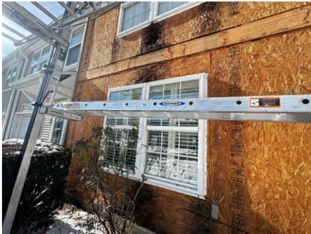
Photo #39: Overview of existing sheathing in poor condition below an upper and a lower window at Unit 33.
