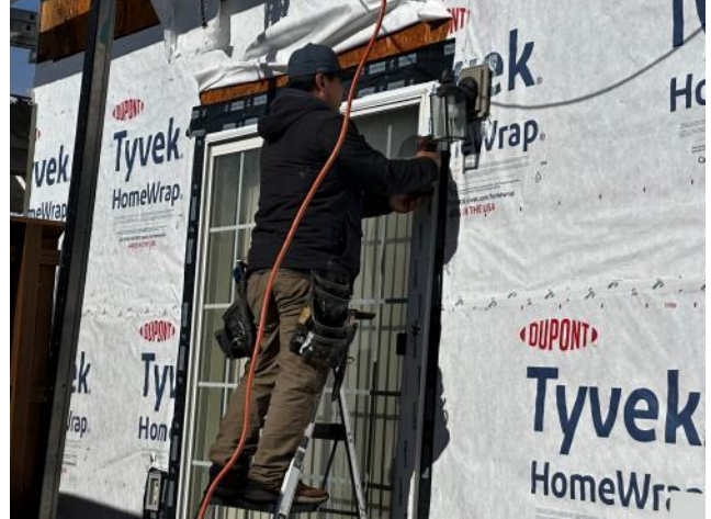
Photo #56: Overview of a sliding door being flashed.
