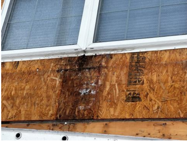
Photo #41: Overview of existing sheathing in poor condition below a box window at Unit 3.
