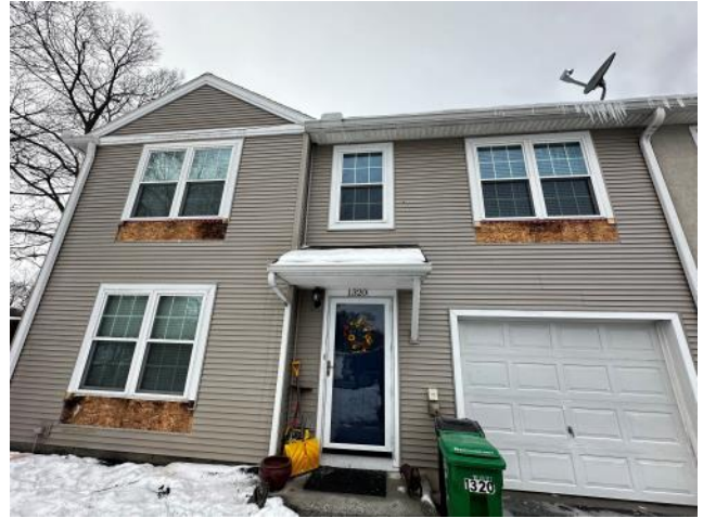
Photo #94: Overview of existing sheathing in poor condition below the front windows at Unit 1320.
