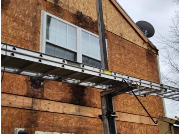
Photo #83: Overview of existing sheathing in poor condition below an upper window at Unit 29.
