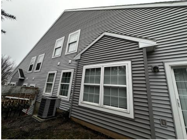
Photo #13: Overview of new vinyl siding installed at a main side of the Building.
