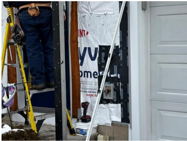
Photo #63: Overview of wall penetrations properly flashed.
