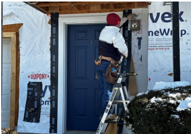
Photo #59: Overview of a front door being flashed.
