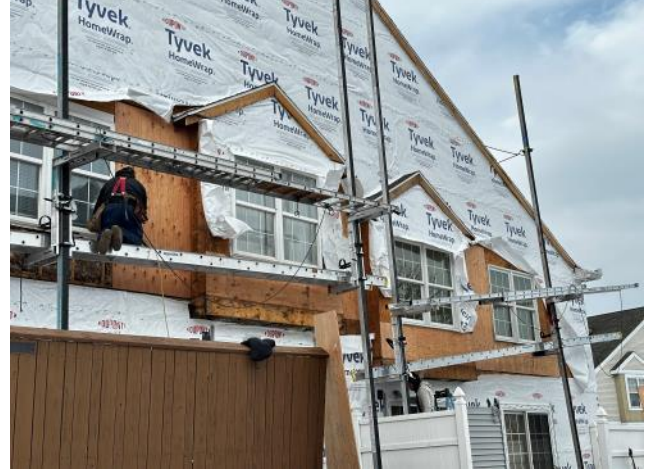
Photo #50: Overview of new sheathing being installed at the box windows.
