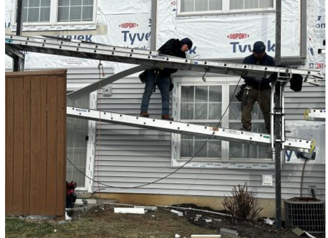
Photo #64: Overview of new vinyl siding being installed at a main side of the Building.
