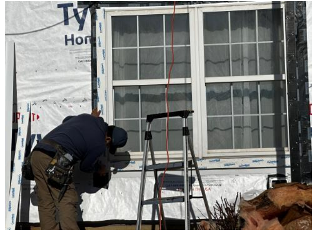
Photo #58: Overview of new pvc trim being installed at a window.
