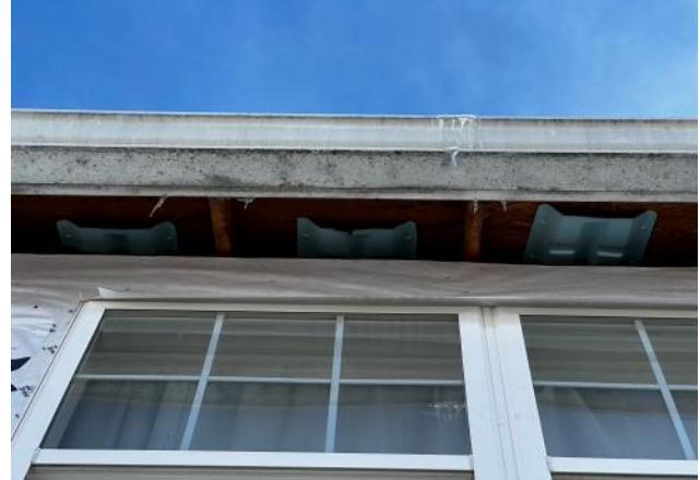
Photo #60: Overview of existing baffles observed in the Building.
