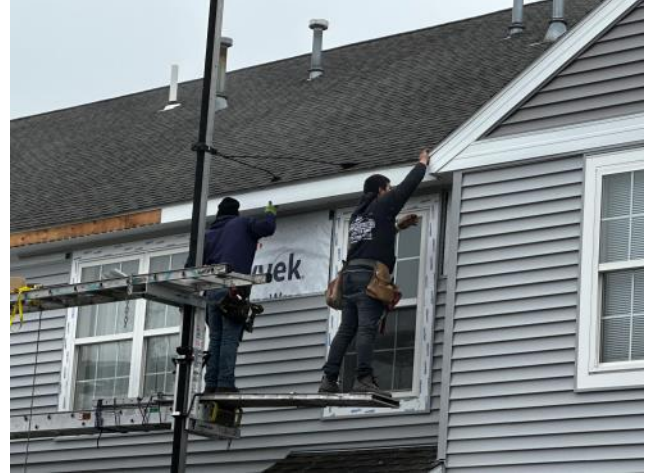
Photo #68: Overview of new metal wrap being installed at a fascia section.
