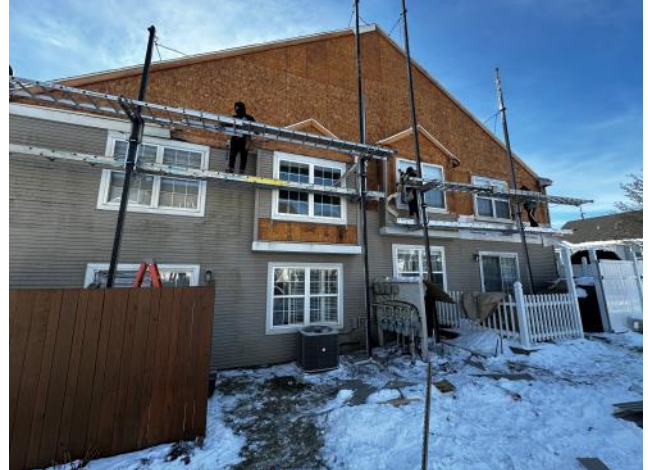
Photo #40: Overview of existing siding/stucco being removed.
