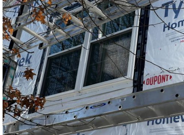
Photo #32: Overview of new metal flashing installed at the bottom of a window and new flashing tape installed at the sides.
