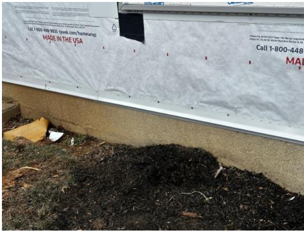
Photo #55: Overview of new starter strip being installed.
