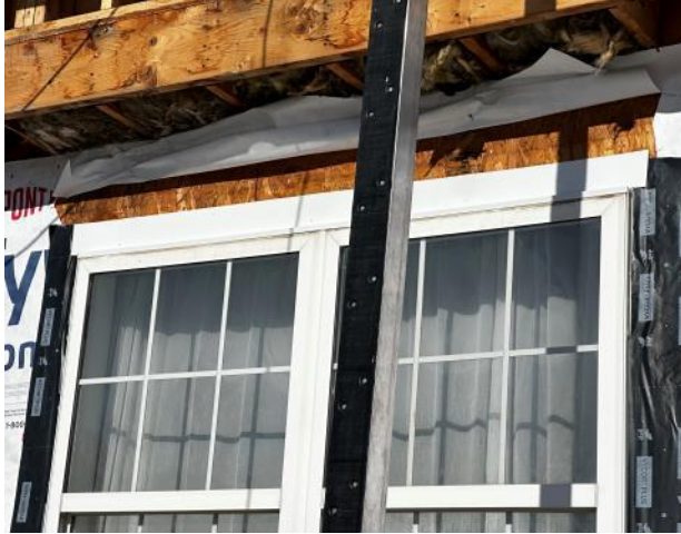
Photo #57: Overview of new metal drip cap being installed on a window.
