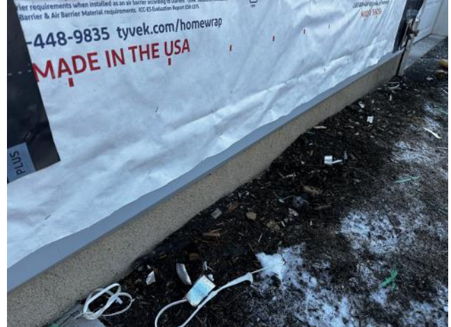
Photo #8: Overview of new starter metal flashing installed.
