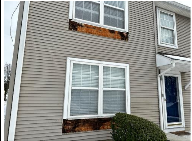
Photo #90: Overview of existing sheathing in poor condition below an upper and a lower window at Unit 2.
