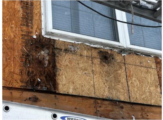
Photo #42: Overview of existing sheathing in poor condition below an upper window at Unit 3.
