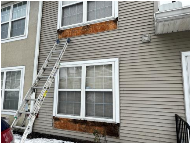
Photo #91: Overview of existing sheathing in poor condition below an upper and a lower window at Unit 6.
