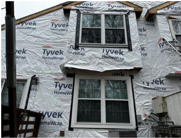
Photo #19: Overview of windows properly flashed and new pvc trim being installed.
