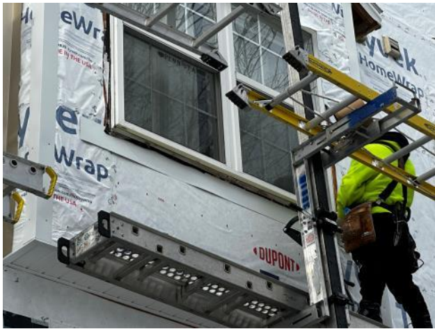
Photo #27: Overview of new metal flashing being installed at the bottom of a window.
