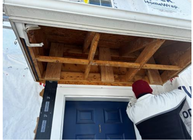
Photo #54: Overview of an entrance roof being reinforced with structural screws in order to eliminate the front brackets.
