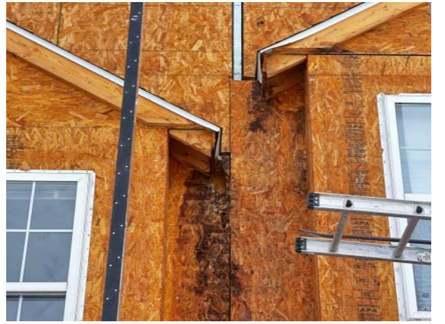
Photo #44: Overview of existing sheathing in poor condition below sections where kick-out flashings are needed.
