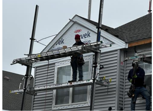
Photo #66: Overview of new vinyl siding being installed at a front small gable.
