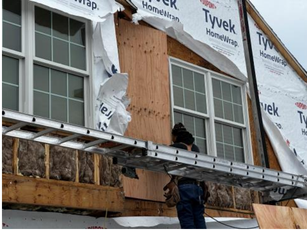
Photo #49: Overview of new insulation and new sheathing being installed.
