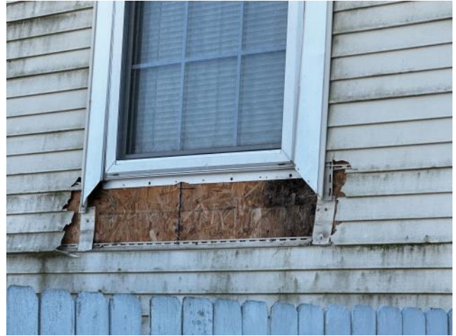
Photo #74: Overview of existing sheathing in poor condition below an upper window at Unit 8.
