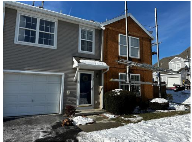
Photo #38: Overview of existing siding being removed. No Water Resistant Barrier was observed.
