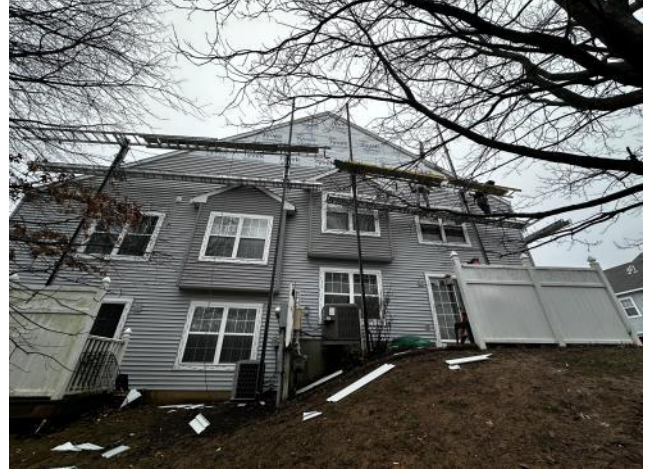
Photo #34: Overview of new vinyl siding being installed at a main side section.
