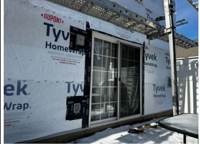
Photo #26: Overview of wall penetrations properly flashed.
