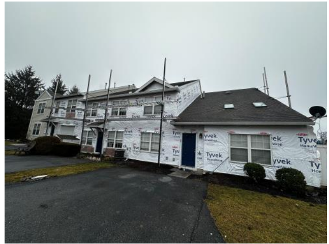
Photo #86: Overview of new Water Resistant Barrier (Tyvek) being installed.
