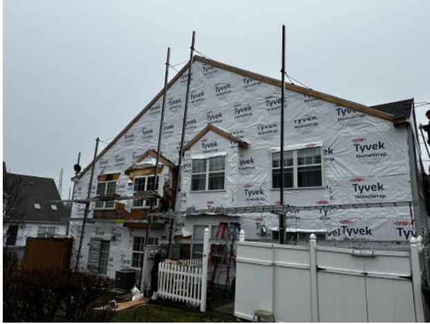
Photo #53: Overview of new Water Resistant Barrier (Tyvek) installed at a main side.
