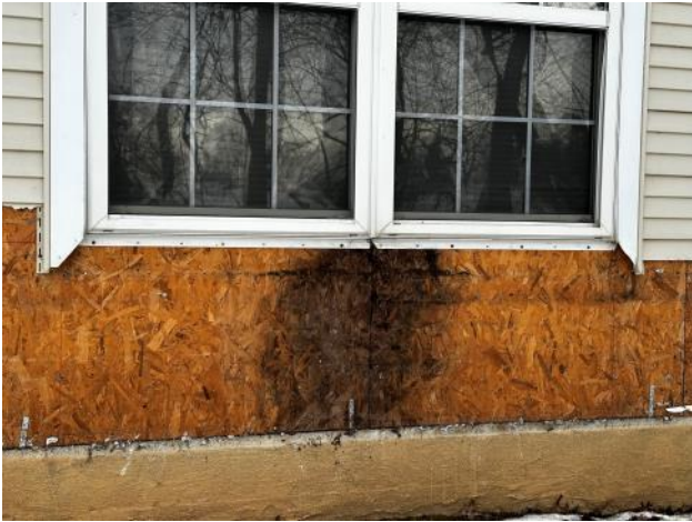
Photo #75: Overview of existing sheathing in poor condition below a box window at Unit 12.
