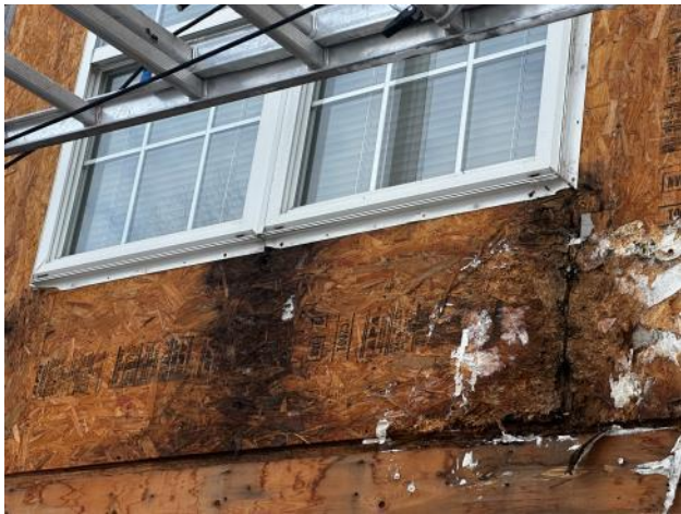
Photo #43: Overview of existing sheathing in poor condition below an upper window at Unit 33.
