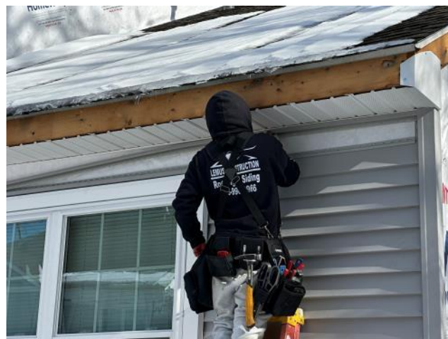
Photo #22: Overview of new intake soffit being installed along new j-channel.
