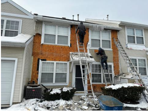
Photo #77: Overview of the demo crew removing the existing stucco at Unit 10.
