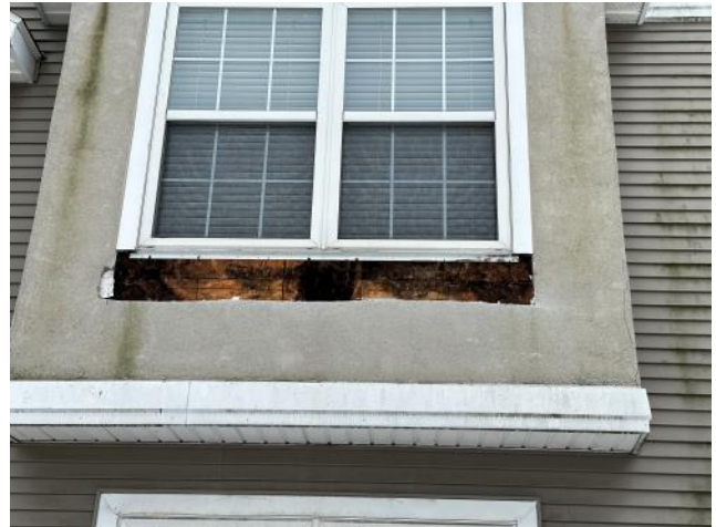
Photo #88: Overview of existing sheathing in poor condition below a box window at Unit 2.
