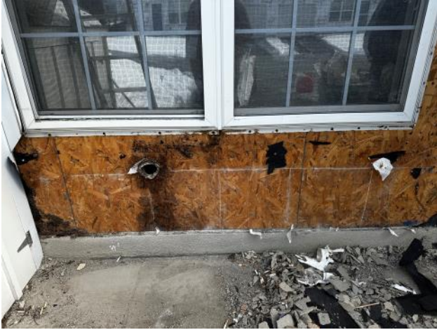
Photo #73: Overview of existing sheathing in poor condition below a lower window at Unit 16.
