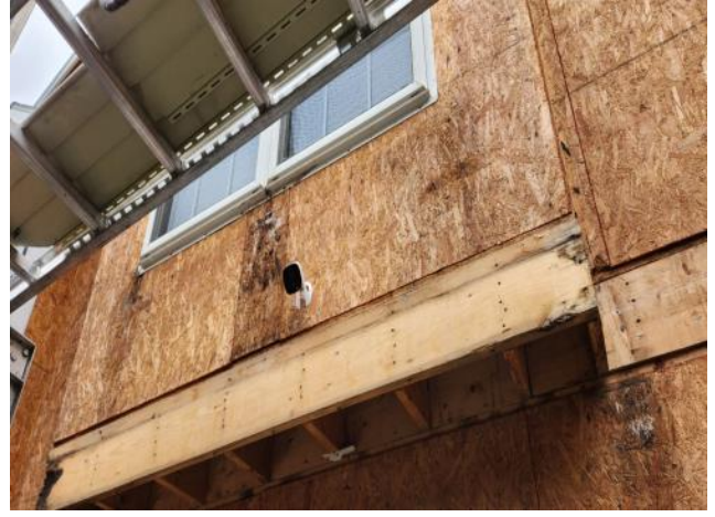
Photo #84: Overview of existing sheathing in poor condition below a box window at Unit 29.
