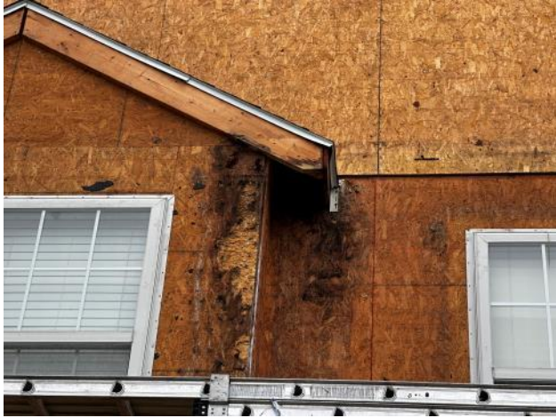
Photo #81: Overview of existing sheathing in poor condition below a section where a kick-out flashing is needed.
