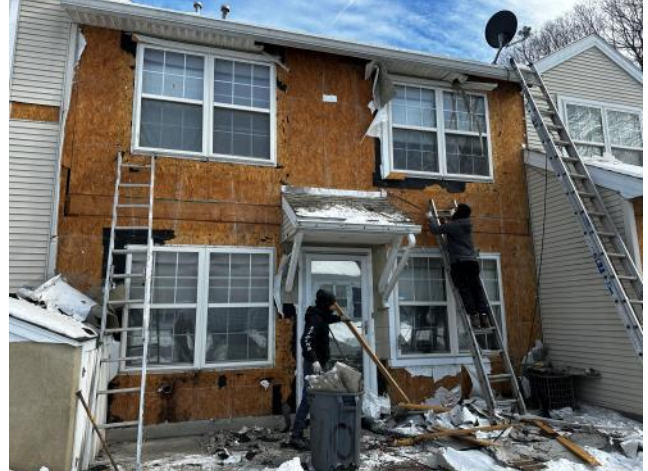
Photo #72: Overview of the demo crew removing the existing stucco.
