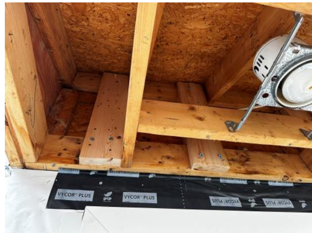
Photo #20: Overview of an entrance roof being reinforced with structural screws in order to eliminate the front brackets.
