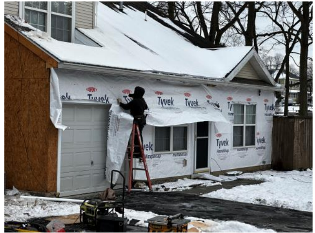
Photo #78: Overview of new Water Resistant Barrier (Tyvek) being installed.
