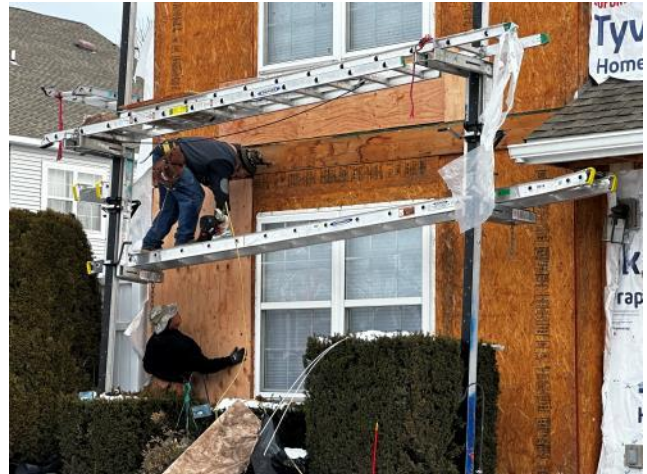
Photo #48: Overview of new sheathing being installed.
