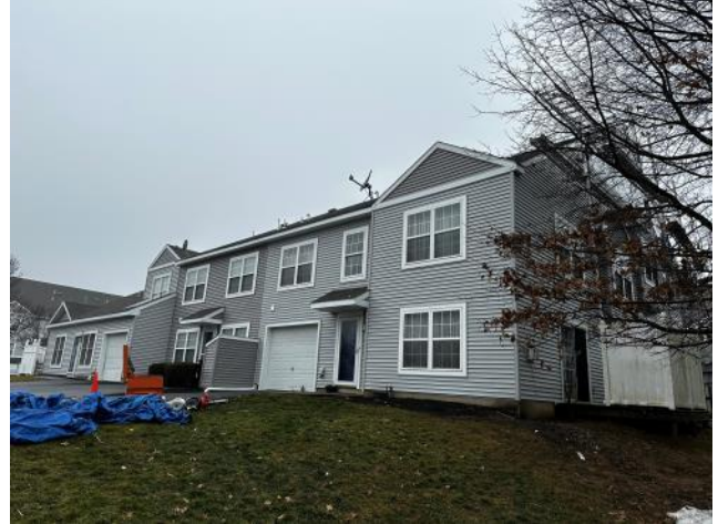
Photo #36: Overview of new vinyl siding completed at a front side of the Building.
