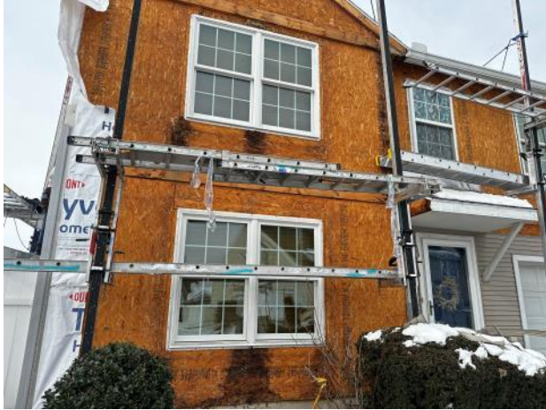
Photo #45: Overview of existing sheathing in poor condition below an upper and a lower window at Unit 31.
