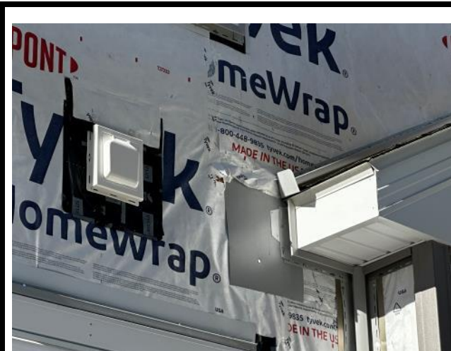
Photo #11: Overview of a new kick-out flashing and metal installed.
