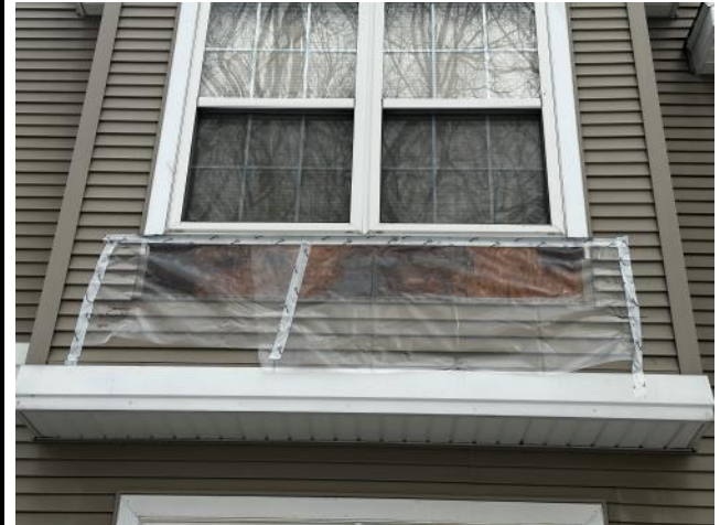
Photo #92: Overview of existing sheathing in poor condition below a box window at Unit 6.
