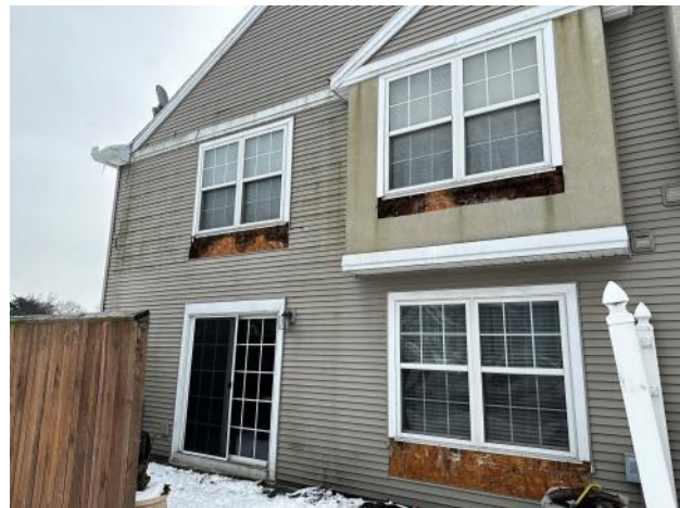
Photo #96: Overview of existing sheathing in poor condition below a box window and an upper window at Unit 1324.
