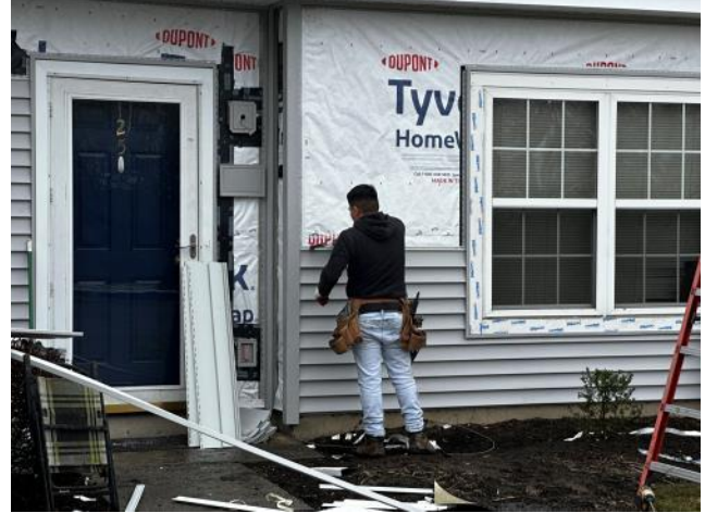
Photo #6: Overview of new vinyl siding being installed.
