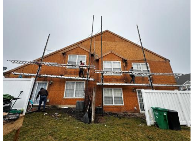
Photo #80: Overview of existing siding/stucco being removed. No Water Resistant Barrier was observed.
