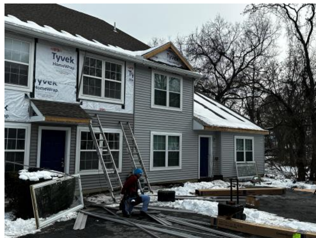
Photo #24: Overview of new vinyl siding being installed at a front section.
