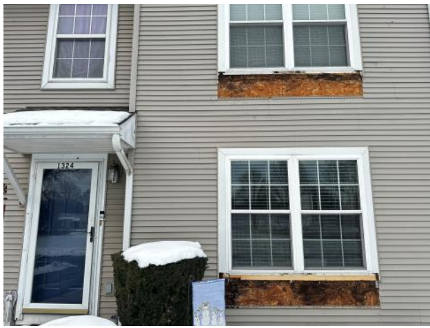
Photo #95: Overview of existing sheathing in poor condition below an upper and a lower window at Unit 1324.
