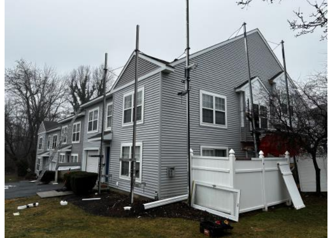
Photo #2: Overview of new vinyl siding being installed at a main side of the Building.
