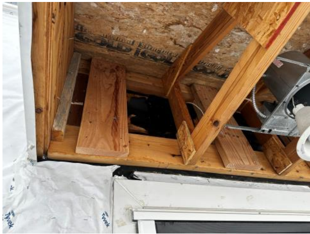
Photo #31: Overview of an entrance roof being reinforced with structural screws in order to eliminate the front brackets.
