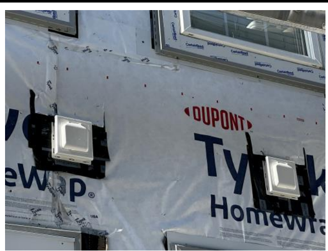
Photo #10: Overview of wall penetrations properly flashed.
