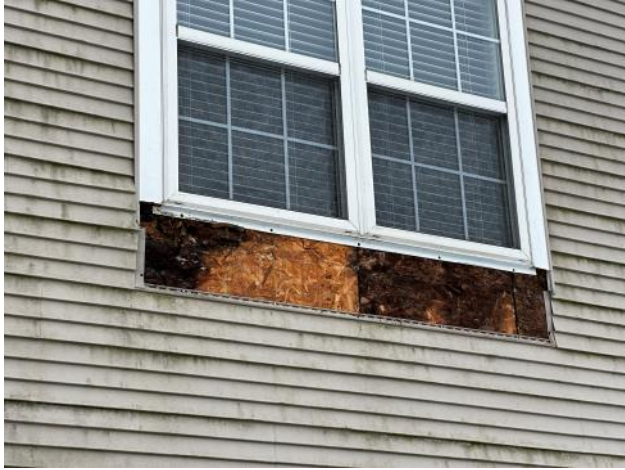
Photo #89: Overview of existing sheathing in poor condition below an upper window at Unit 2.
