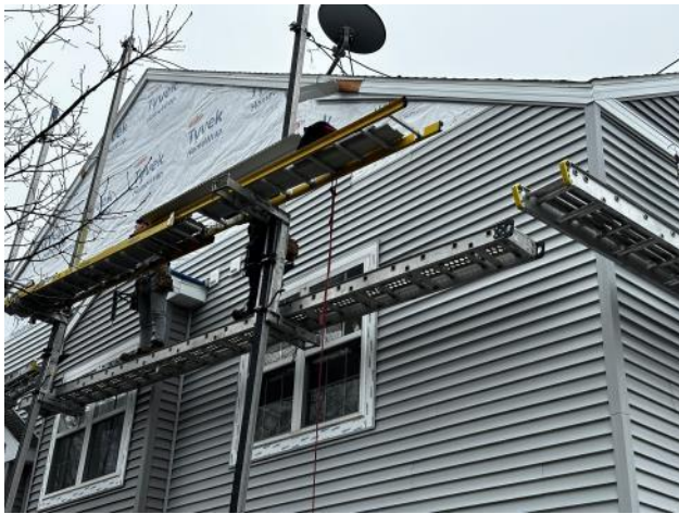
Photo #35: Overview of new vinyl siding being installed.
