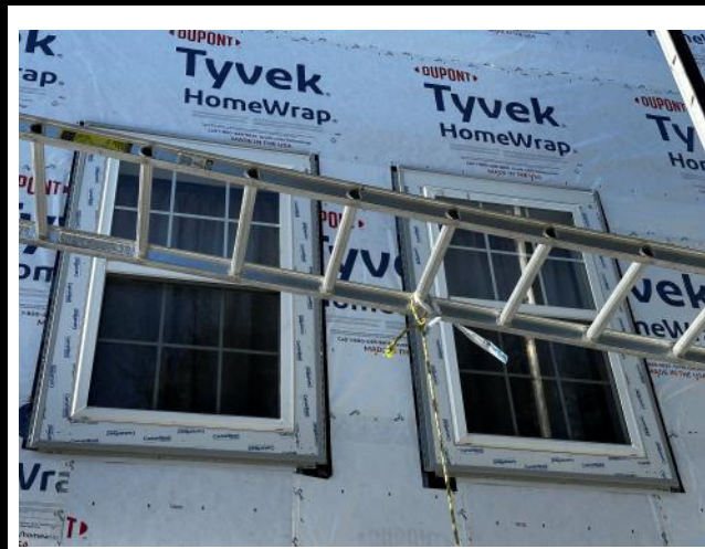
Photo #9: Overview of new pvc trim installed at two windows.
