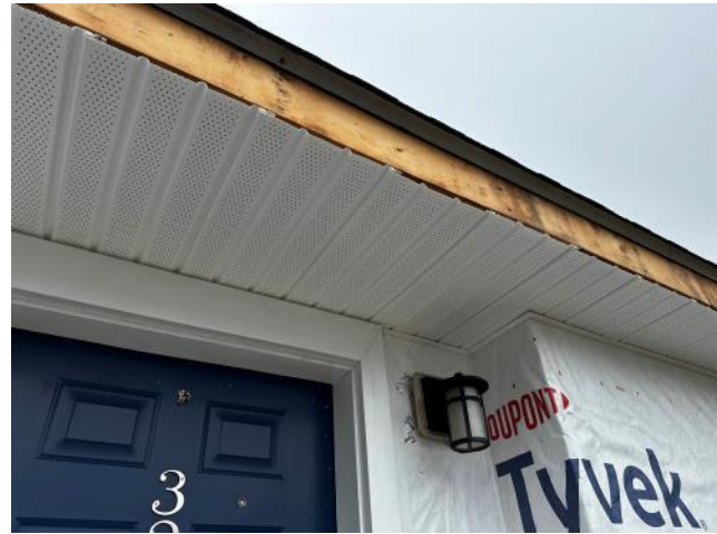
Photo #18: Overview of new intake soffit being installed.
