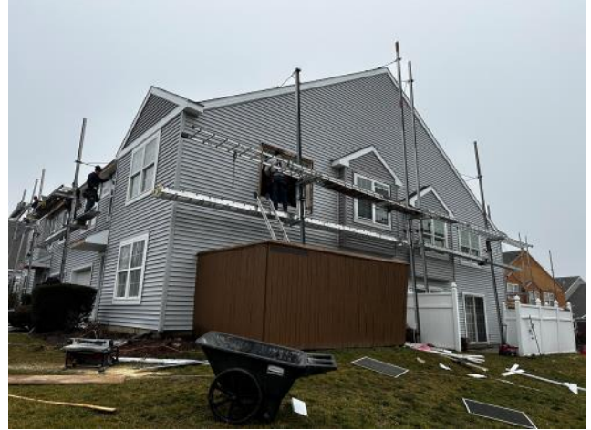
Photo #70: Overview of new vinyl siding being installed at a main side section.
