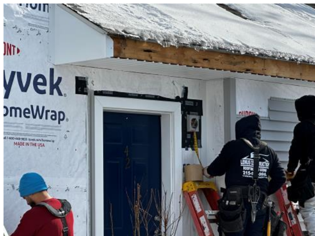
Photo #23: Overview of wall penetrations properly flashed.
