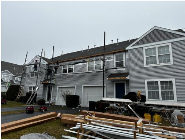
Photo #69: Overview of new vinyl siding being installed at a front section.
