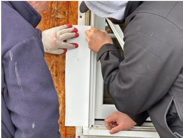
Photo #47: A custom flange had to be installed in order to properly flash this type of window.
