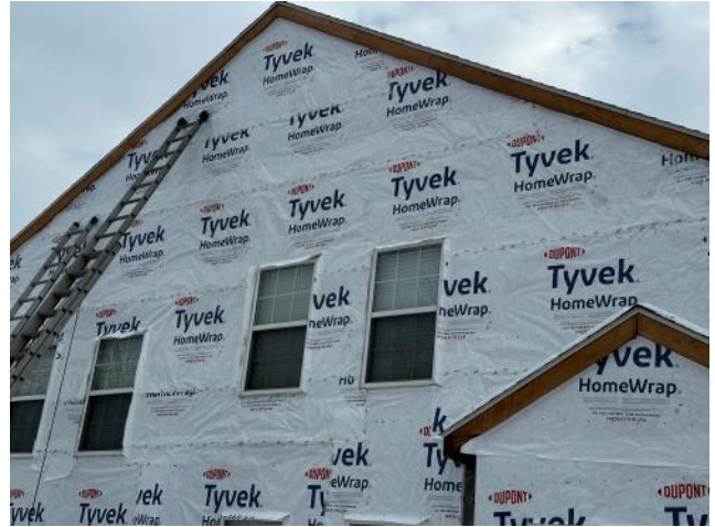
Photo #54: Overview of new Water Resistant Barrier (Tyvek) being installed at a main side of the Building.
