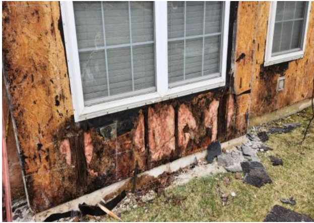
Photo #49: Overview of existing sheathing in poor condition below a box window at Unit 20.
