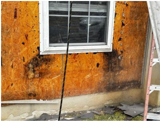
Photo #51: Overview of damaged sheathing below a lower window at Unit 26.
