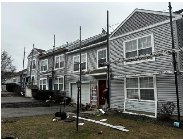
Photo #7: Overview of new vinyl siding being installed at a front of the Building.
