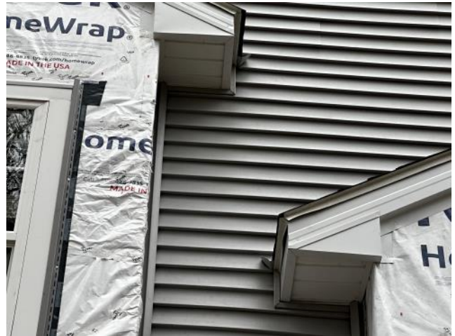
Photo #4: Overview of new kick-out flashings installed.
