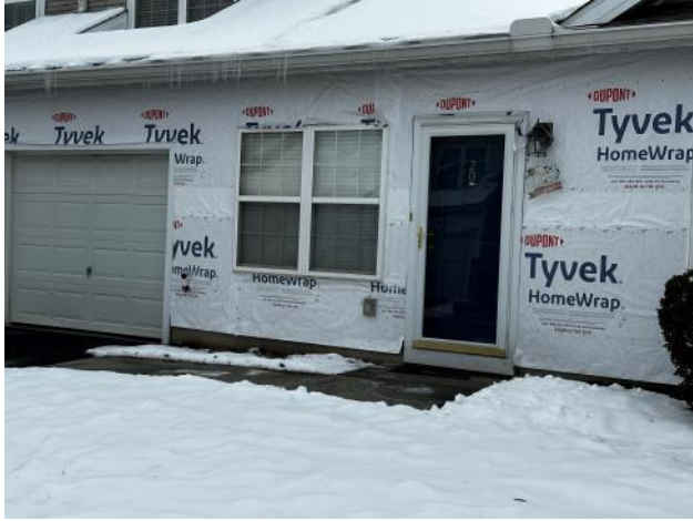
Photo #53: Overview of new Water Resistant Barrier (Tyvek) being installed at the other front side of the Building.
