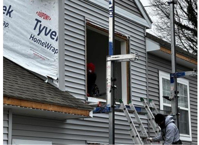
Photo #6: Overview of a window opening getting ready before installing the new window.
