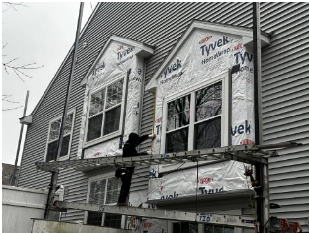
Photo #3: Overview of new vinyl siding being installed the box windows.
