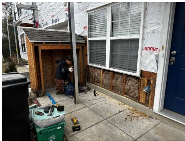
Photo #30: Overview of new insulation and new sheathing being installed.
