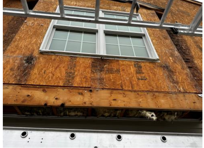
Photo #42: Overview of damage sheathing below a box window at Unit 31.
