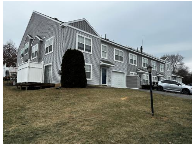
Photo #12: Overview of new vinyl siding completed at a front and side of the Building.
