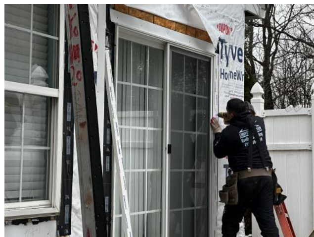
Photo #22: Overview of new vinyl siding being installed at the other front section.
