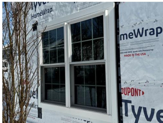
Photo #28: Overview of new pvc trim installed at another window.
