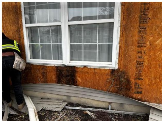
Photo #39: Overview of damaged sheathing below a lower window at Unit 1.
