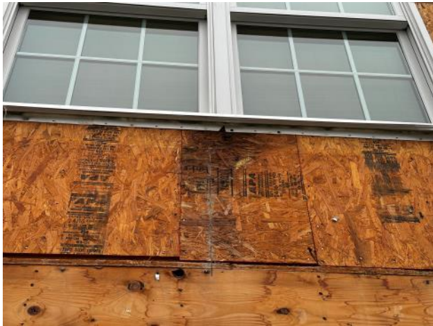
Photo #43: Overview of damage sheathing below an upper window at Unit 31.
