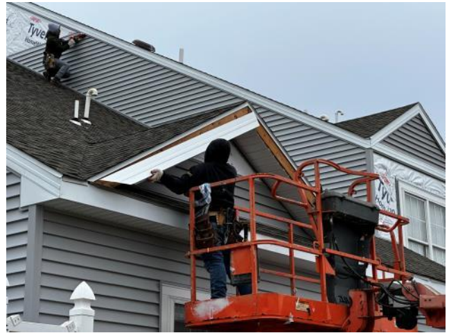
Photo #34: Overview of new metal wrap being installed at the rake boards at a front gable
