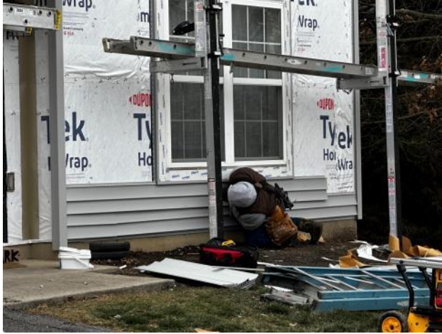
Photo #33: Overview of new vinyl siding being installed.
