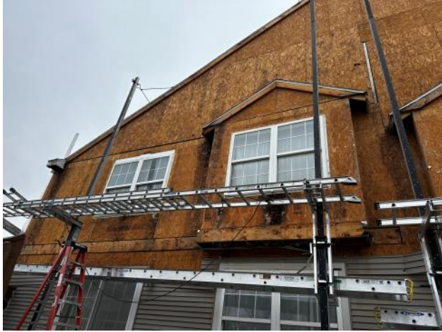
Photo #41: Overview of damage sheathing below an upper window and a box window at Unit 1.
