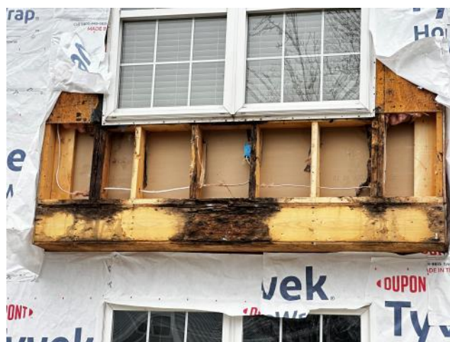
Photo #24: Overview of box window at Unit 32. Framing was starting to get severely damaged. Lemus replaced/reinforced studs and 2x10 accordingly.
