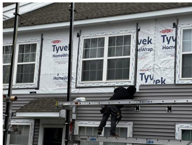
Photo #10: Overview of new vinyl siding being installed. Siding installation was being completed on this Building 18.
