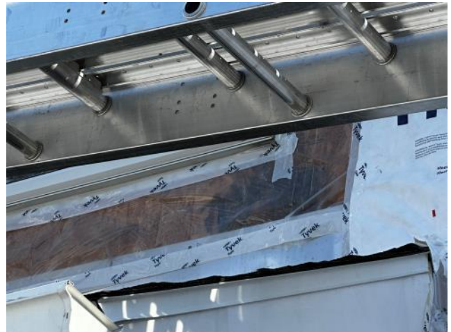
Photo #46: Overview of damage sheathing below another upper window at Unit 3.
