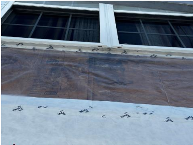
Photo #45: Overview of damage sheathing below an upper window at Unit 3.
