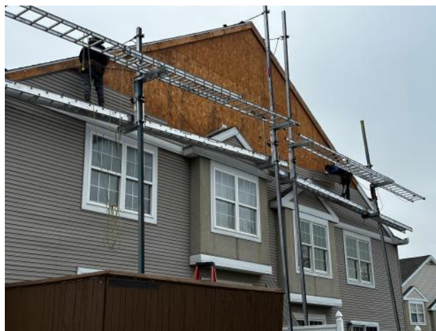
Photo #38: Overview of existing siding being removed. No Water Resistant Barrier was observed behind the existing siding.
