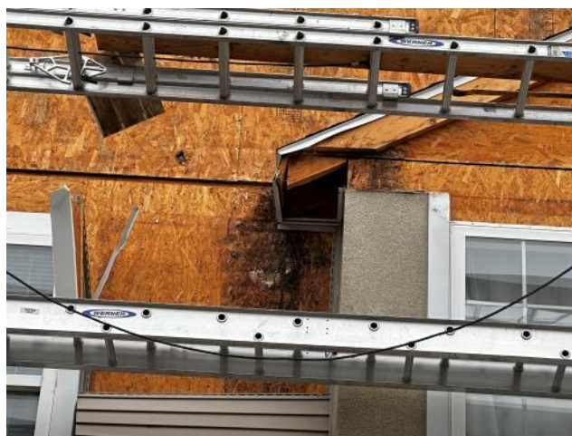
Photo #40: Overview of damaged sheathing where a kick-out flashing was missing.
