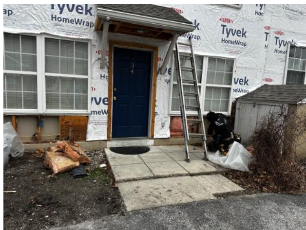
Photo #25: Overview of existing insulation and damaged sheathing being replaced.
