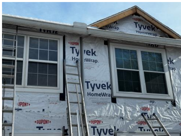
Photo #27: Overview of windows properly flashed and new pvc trim being installed.
