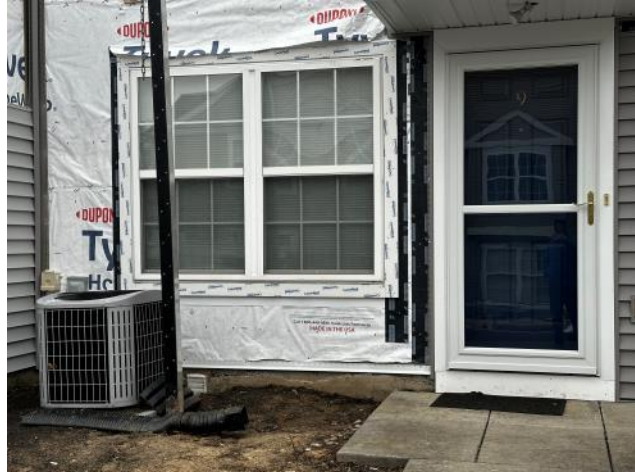
Photo #32: Overview of new starter strip installed.
