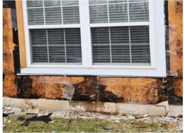
Photo #50: Overview of existing sheathing in poor condition below a box window at Unit 26.
