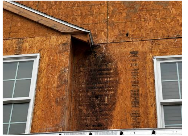
Photo #44: Overview of damaged sheathing where a kick-out flashing was missing.
