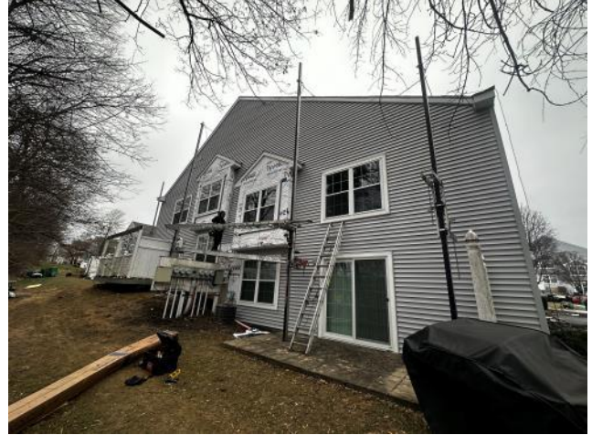
Photo #2: Overview of new vinyl siding being installed at a main side of the Building.
