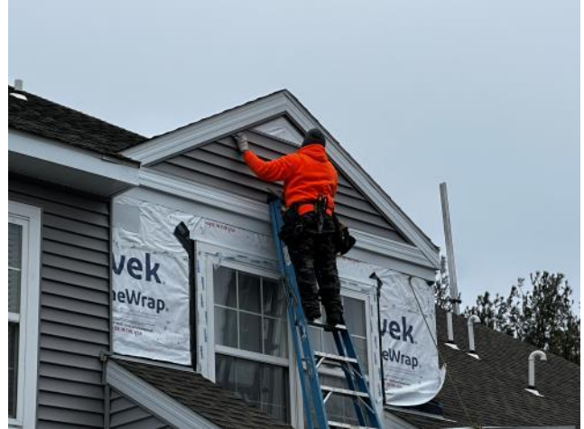
Photo #16: Overview of new vinyl siding being installed at a front gable.
