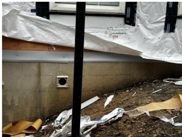
Photo #17: Overview of new metal wrap at the rake board and new vinyl siding being installed at a front gable.
