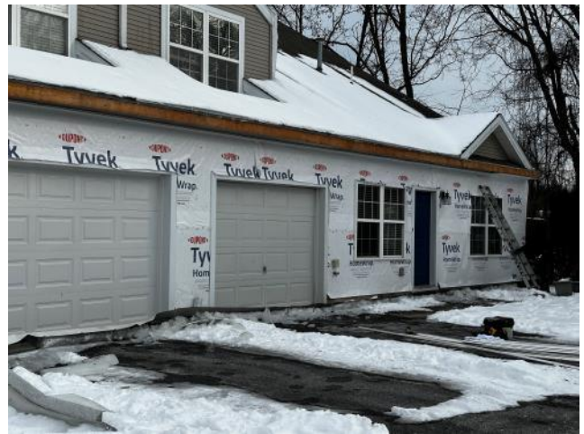
Photo #52: Overview of new Water Resistant Barrier (Tyvek) being installed at a front side of the Building.
