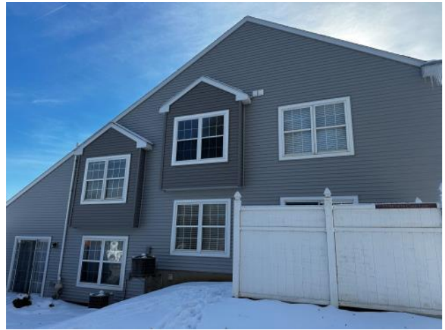
Photo #14: Overview of new vinyl siding completed at the main side of the Building.
